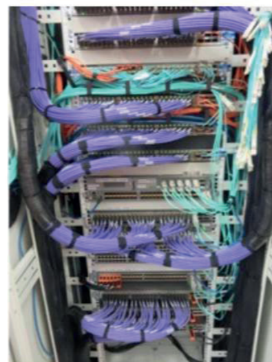
...and after the work.
